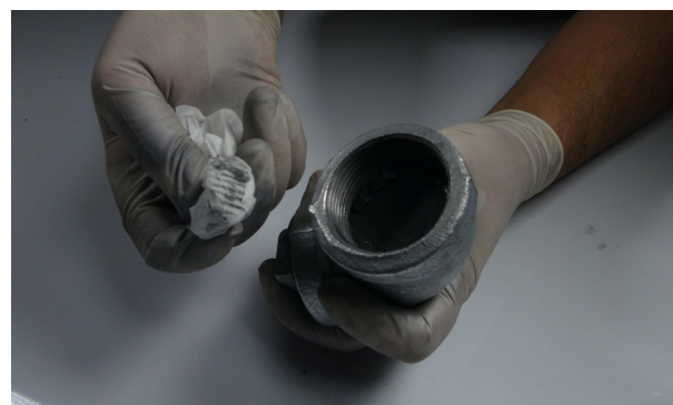
6. Wipe the internal screw thread with a cloth so as not to ignite the fireworks while sealing the pipe.
